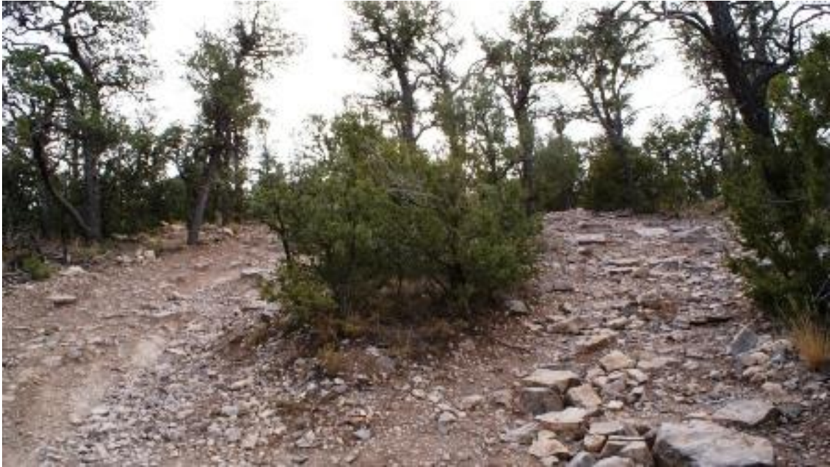
One of the 5 sections of the road with alternate routes.
