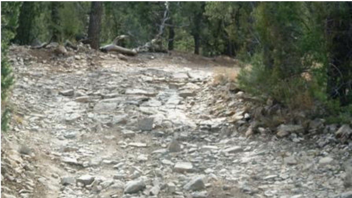
Most of FR13 is cobble stone and loose rocks.
