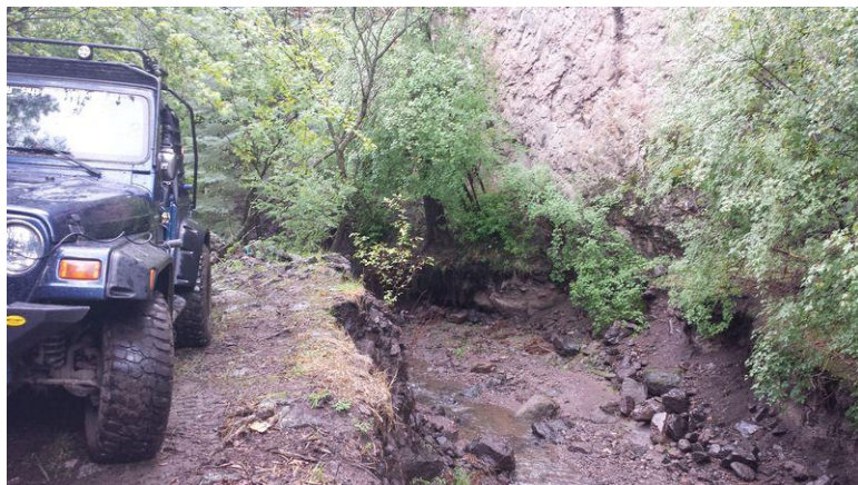
Above the winch point where the bank collapsed. Everything between driver's side rear wheel and edge of the bank is now gone!
