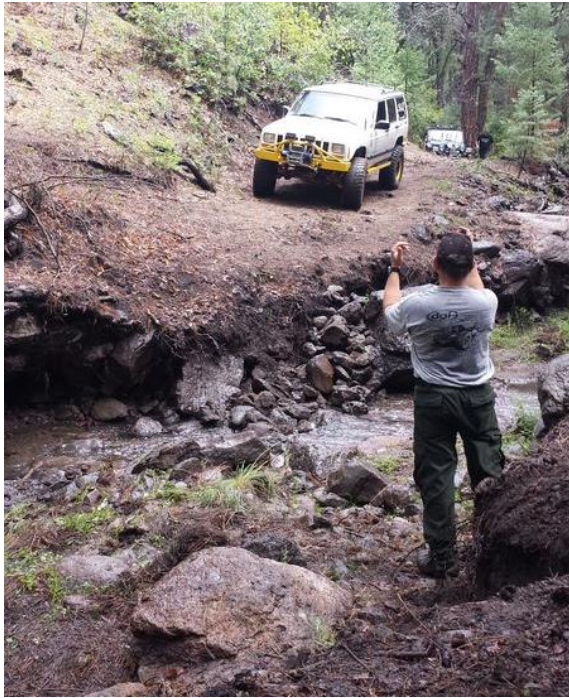
Descending the rebuilt trail the next day. All of the rock in the picture was filled in by hand.
