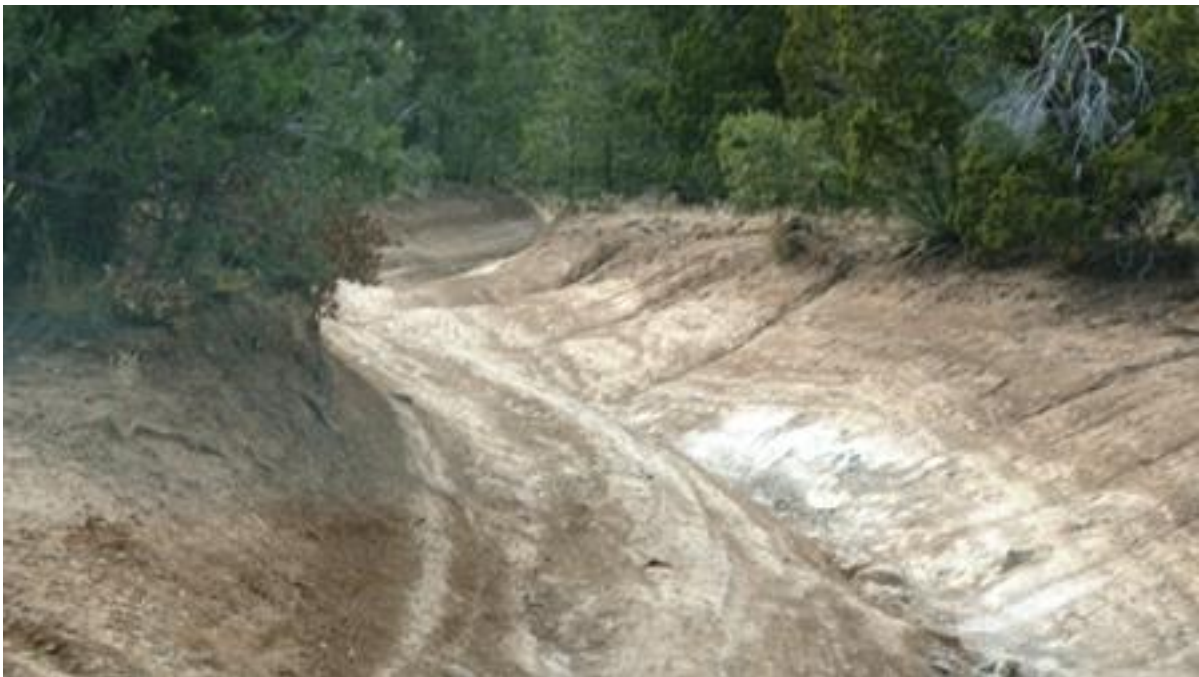
Parts of FR13 look like this, luckily was dry that we could straddle the ditch.
